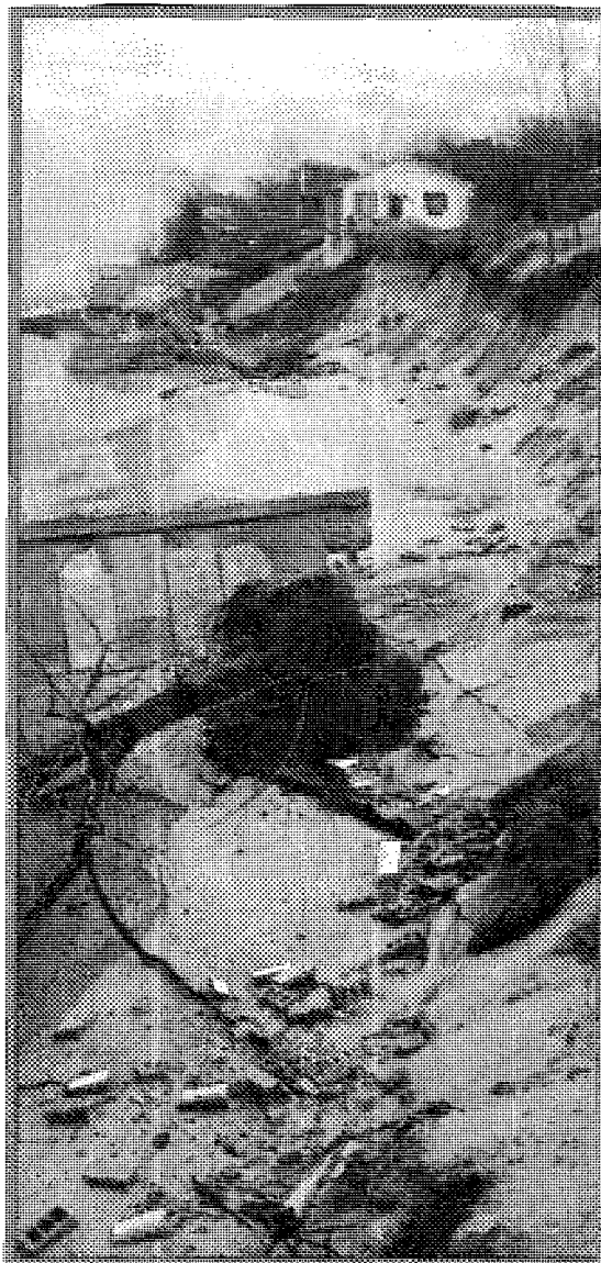
High lake levels and severe weather conditions can cause damage to unprotected properties. Above, shoreline damage to the southern shore of Lake Michigan.
